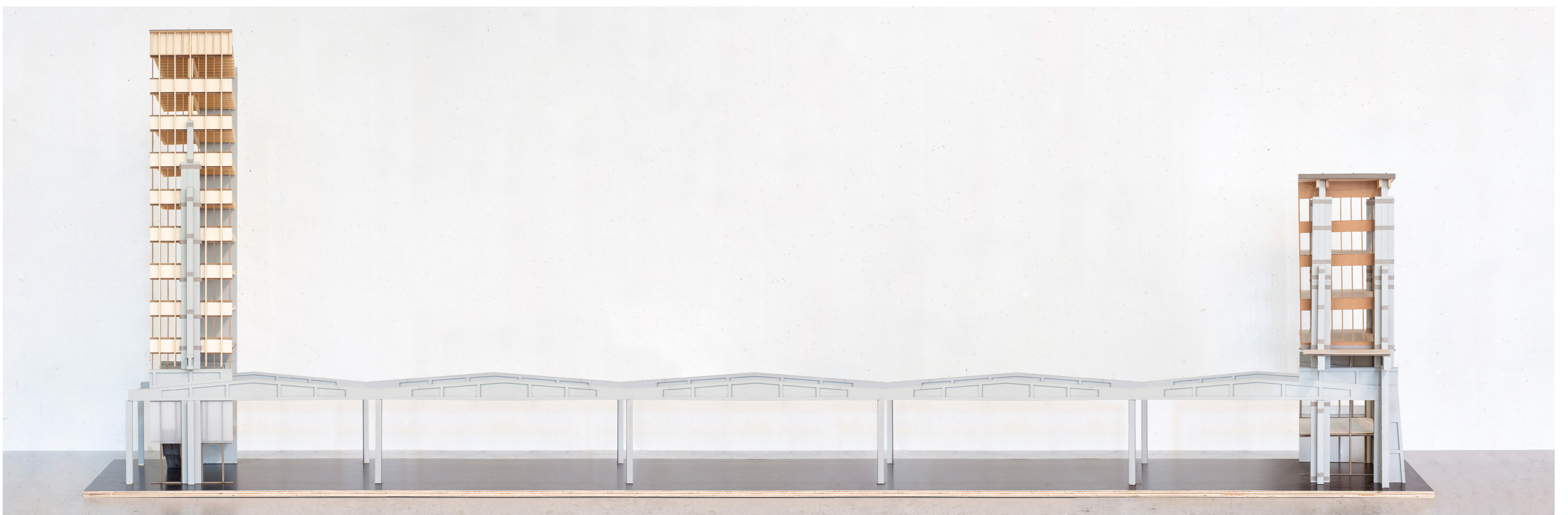
1:50 model, showcasing how the two sections of the new building relate to the old structure they are built on top of.
